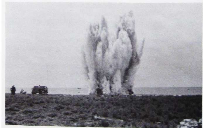
Figure 11. UDT blasting coral heads from beaching area. Howland Island (US Atomic Energy Commission 1963).
